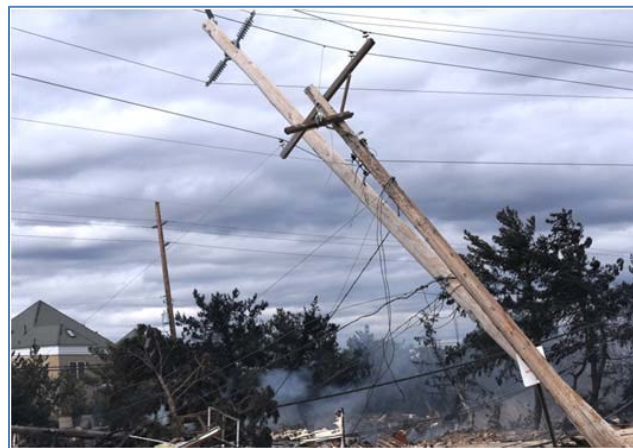
Figure 2-3 Extensive power line damage during Superstorm Sandy (courtesy NJ Task Force 1, 2012).
